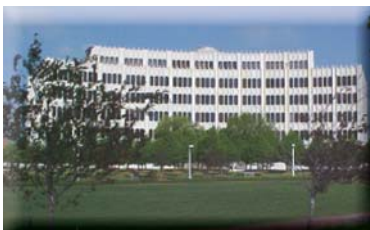
Connors Building Current Rating: 83 (+5)
